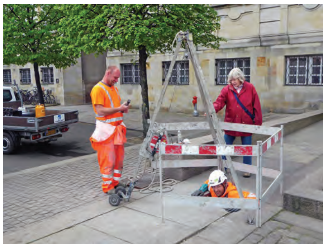
Maintenance gang inspecting the sewers and escape tunnel beneath the Christiansborg Palace. Photo Martin Dixon
